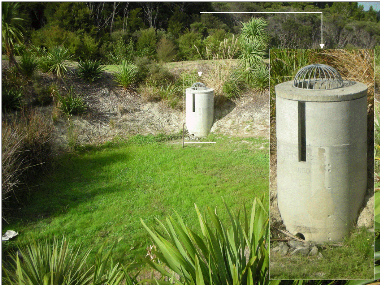
Figure 2: General View of Original Pond Looking South West with Close-up of Outlet
