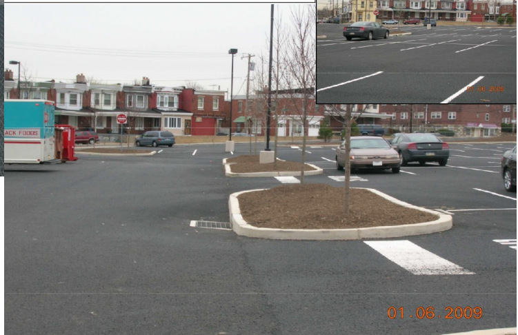
Finished parking lot on top of RainTank™ System
