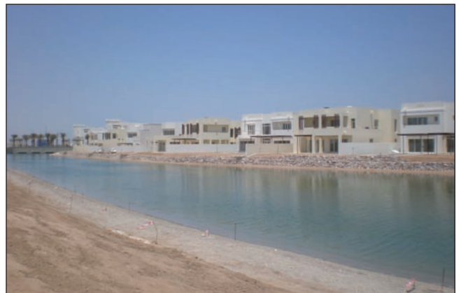
Canal 3 ® covered with soil WAVE Project, Muscat, Oman
