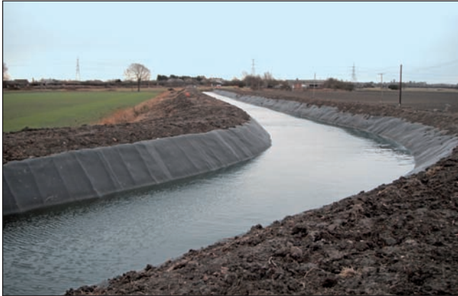
Canal 3 ® exposed application Soham Lode Project, Soham, United Kingdom
