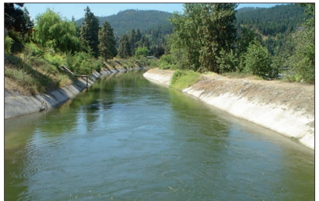
Canal 3 ® covered with shotcrete Dryden Canal Project, Wenatchee, Washington, USA
