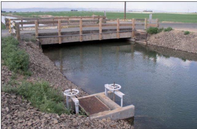
Canal 3 ® covered with gravel Quincy Project, South Columbia, Washington, USA
