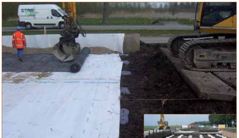
Piled embankment, Project: N210, NL
