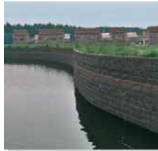
Segmental Retaining walls
