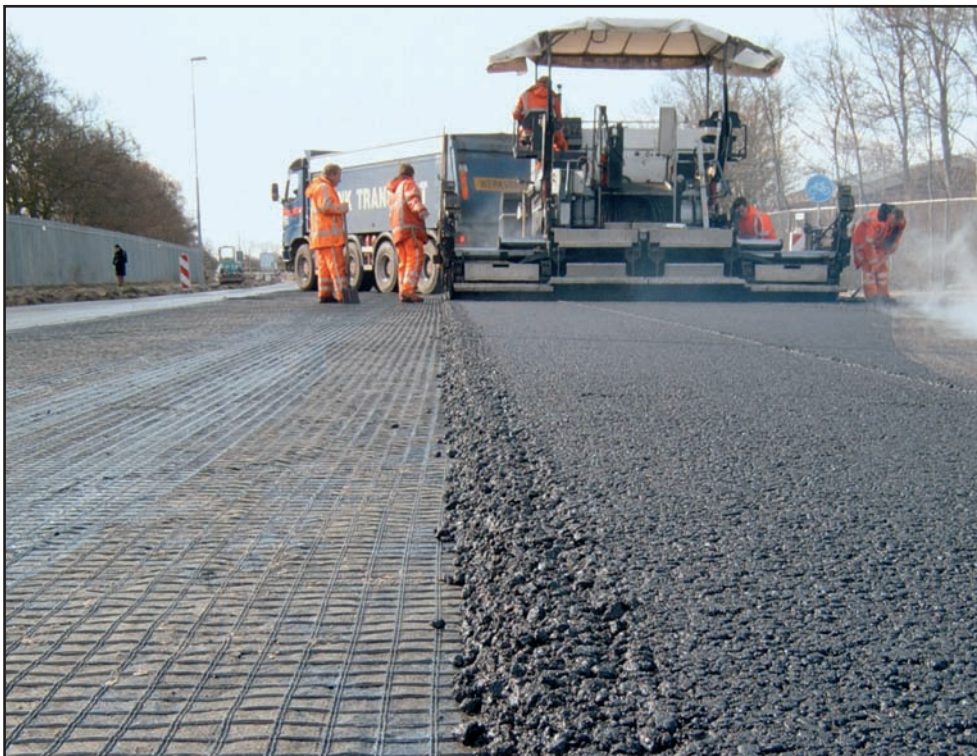
Installation of HaTelit® in the Netherlands
