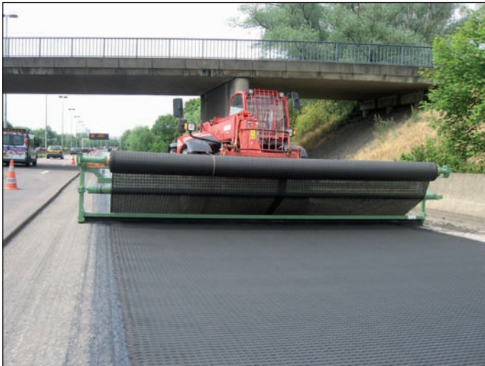
Mechanical installation using large unrolling device
