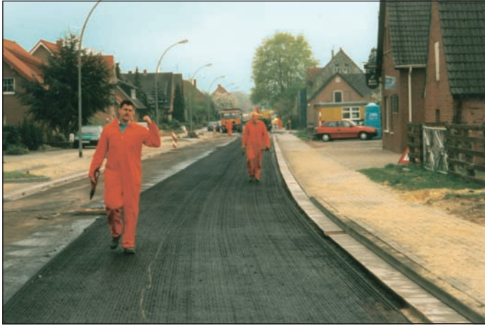
Installation of HaTelit ® in Ochtrup, Germany, 1996
