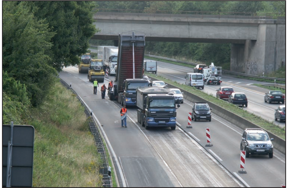
Installation of HaTelit® in Germany
