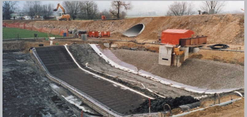
Settlement lagoons - Lining with NaBento®
