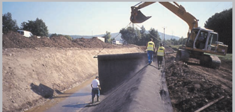
River-bed lining with NaBento®
