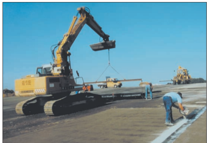
NaBento®- installation in a landfill construction
