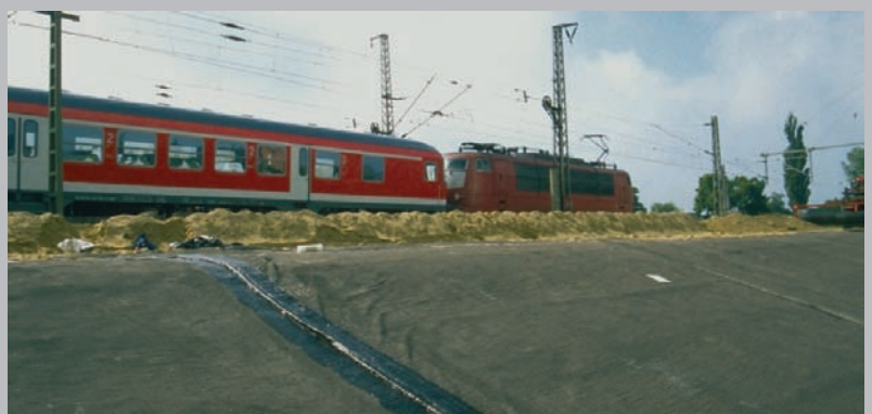
Railway lining with NaBento®
