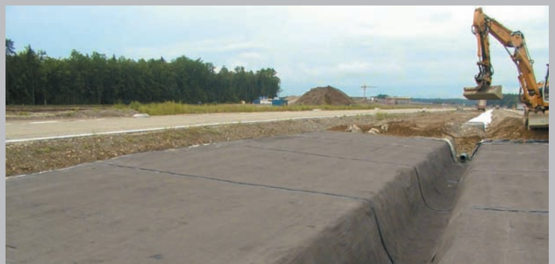
Groundwater protection on a road scheme
