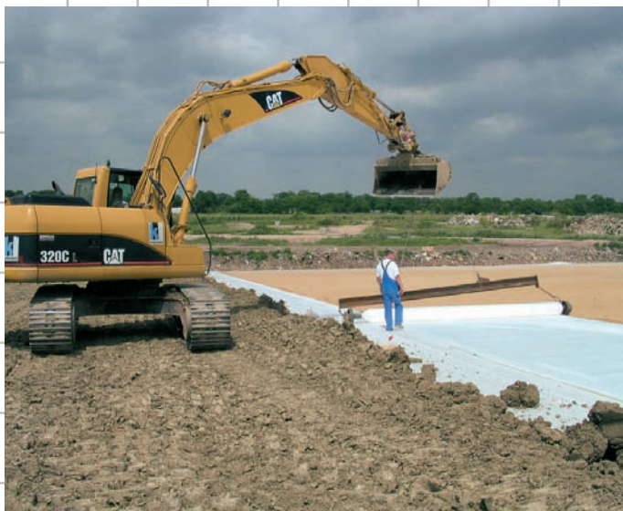
Capping a sludge lagoon
