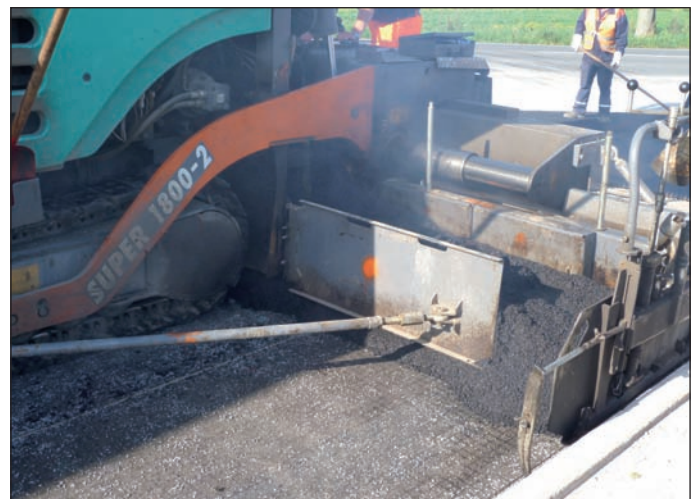
Asphalt installation on SamiGrid®
