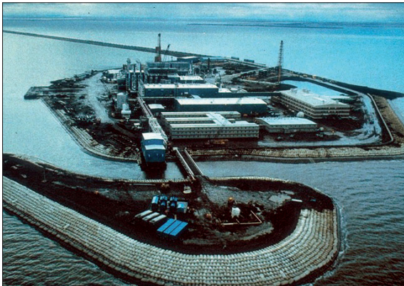
Endicott Island after completion of work in 1985
