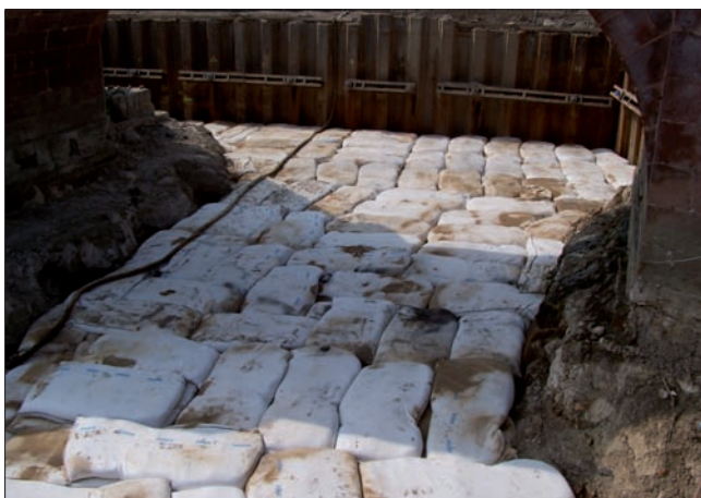
SoilTain ® bags as scour protection for a bridge pier
