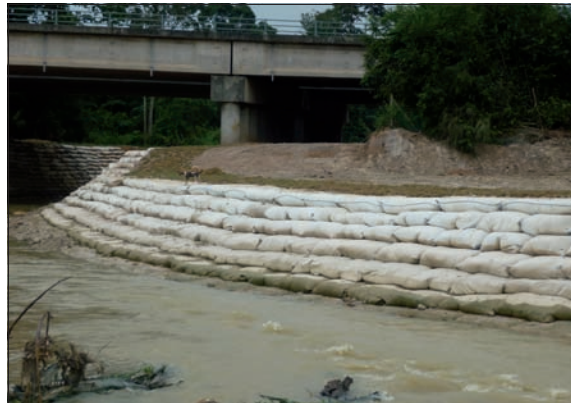
Sungai Melaka project, Malaysia in 2011
