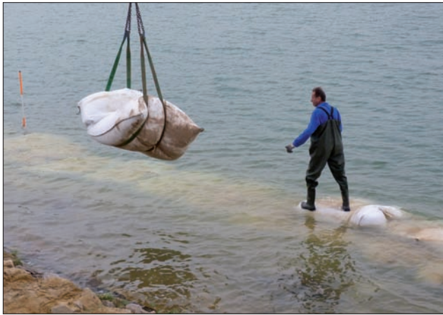
Placement of the SoilTain ® Bag
