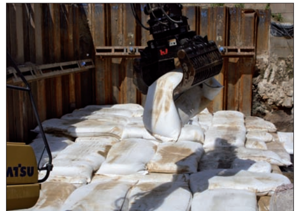
Fig. 6: Placement of the SoilTain® Bags
