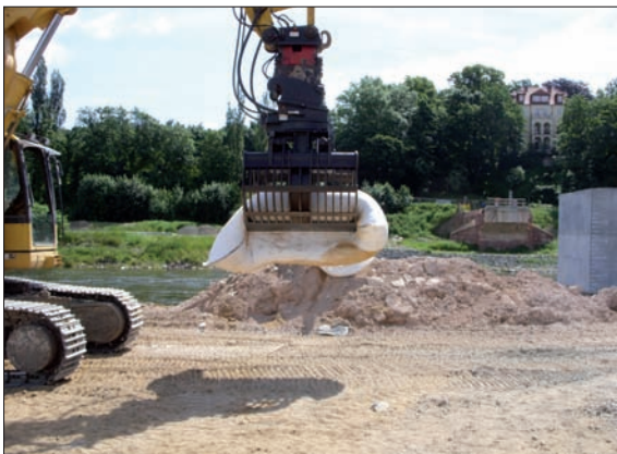
Fig. 5: Transportation by an excavator with a grab
