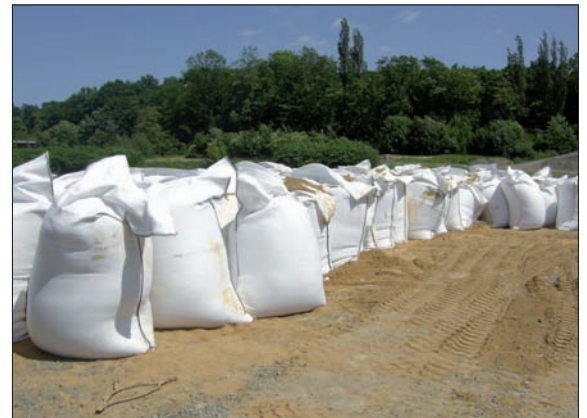
Fig. 4: Prepared SoilTain® bags, waiting for installation
