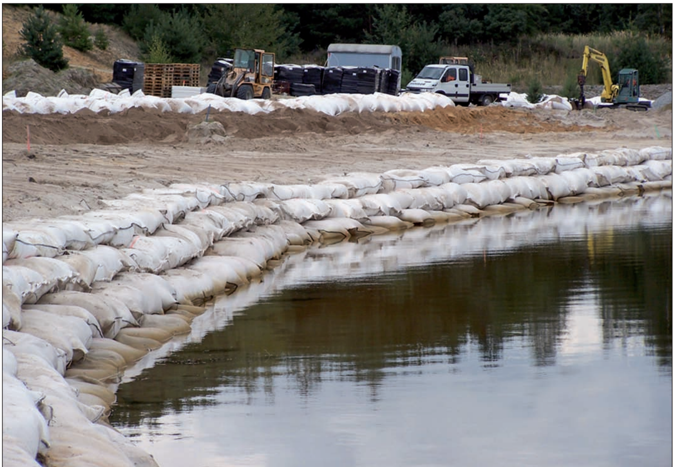
Overview of a typical SoilTain® bag construction site
