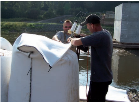
Fig. 3: Closing of the SoilTain® Bags with a hand-held sewing machine
