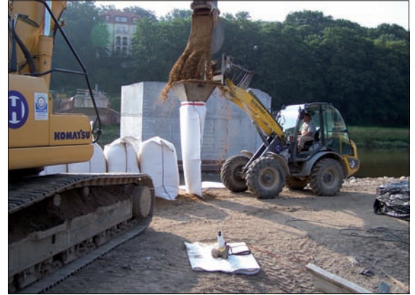
Fig. 2: Filling process of the SoilTain® Bags with a funnel
