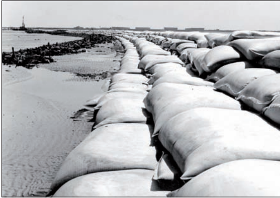
Construction of the dike core at the Rüstersieler Watt 1963
