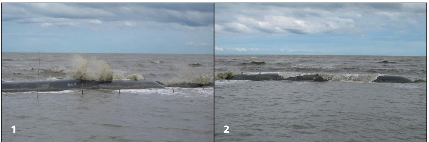
Picture 1/2: SoilTain® Tubes as breakwaters temporarily protruding from the water under wave action during low tide
