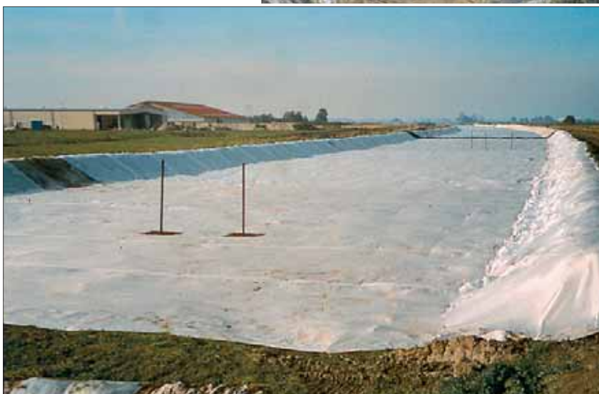
reinforcement with Stabilenka® 300/45 for the bypass embankment
