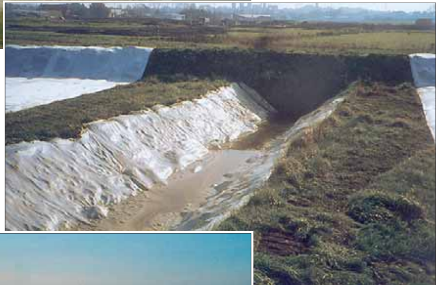
additional reinforcement to existing trenches
