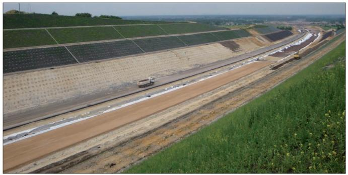
Fig. 13: Fortrac 3D<sup>®</sup> slope reinforcement in cut section
