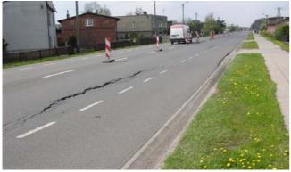
Fig. 4: Surface deformation due to mining activity, DK 44, Poland
