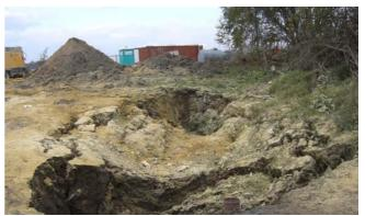
Fig. 7: Sinkhole forming during construction
