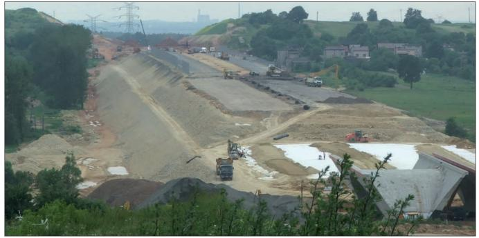
Fig. 15: Fill section of highway embankment
