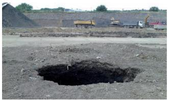
Fig. 6: Sinkhole forming during construction
