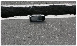
Fig. 5: Deformations forming differential movements, DK 44 Poland
