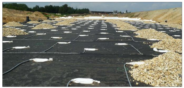
Fig. 11: 2<sup>nd</sup> Monitoring system on Fortrac® geogrid, System NeoStrain®
