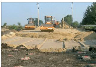
Cut off vibro columns in piled foundation and incorporation of mixed aggregate layer
