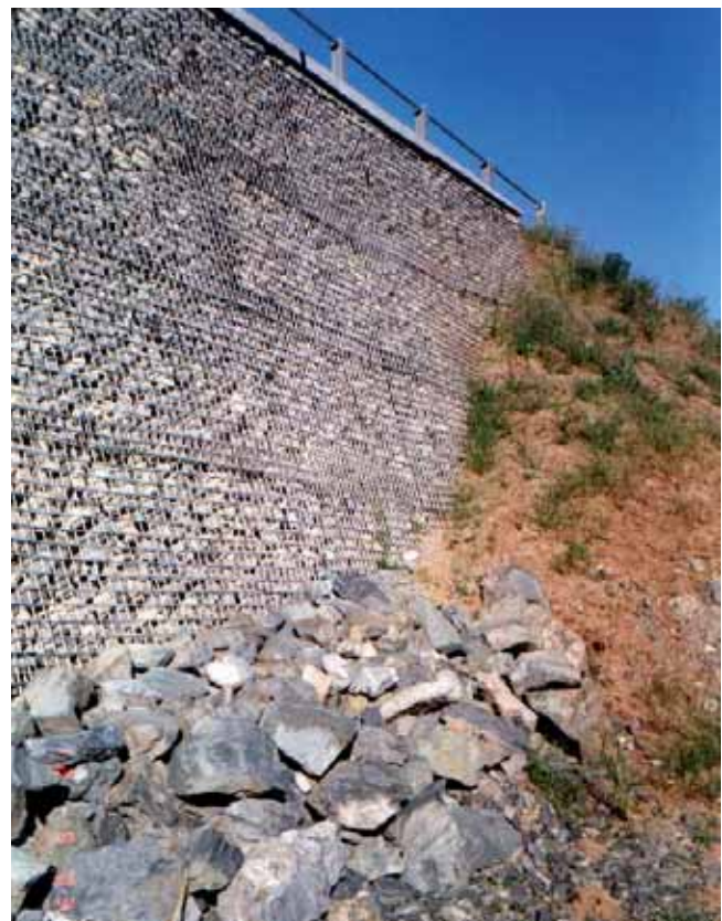
The finished Muralex® facing using stone fill
