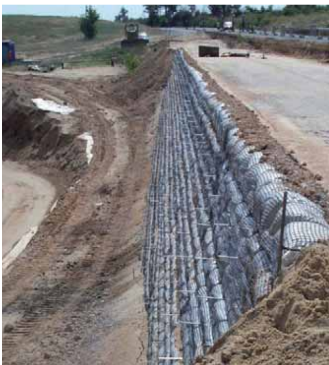
Reinforced soil block using sandbag formers
