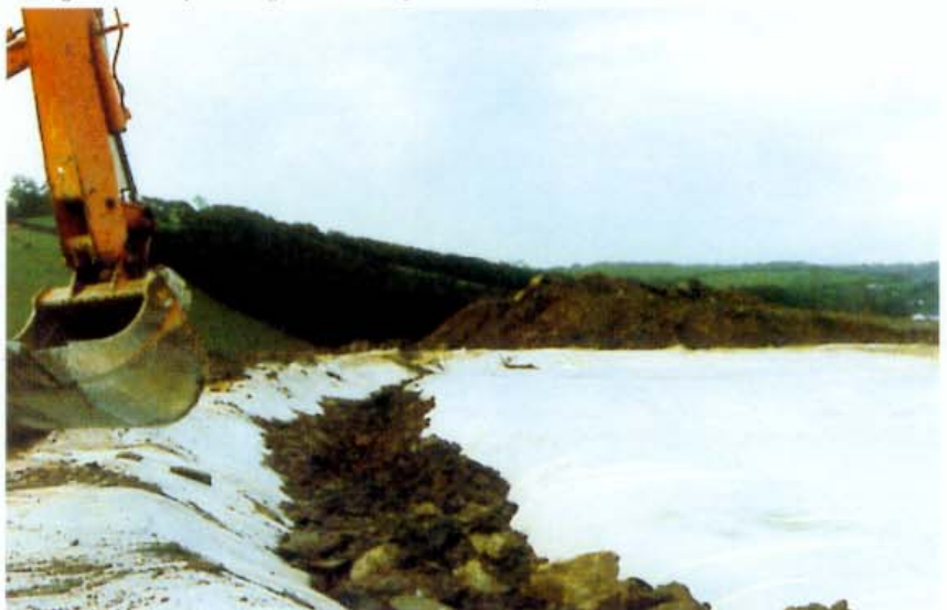
After the fabric had been installed, a 'sludge lock' was created to prevent sludge from squeezing out during initial fill placement.
