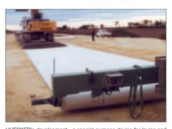
HUESKER's development - a special-purpose device for laying and pre-tensioning **Stabilenka**® 1000/100
